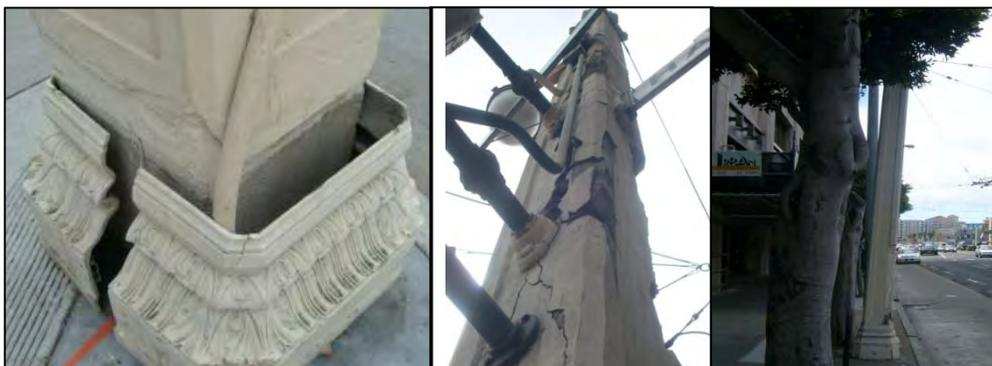
**Photos 31-33. Damaged and leaning OCS support pole/streetlights.**
