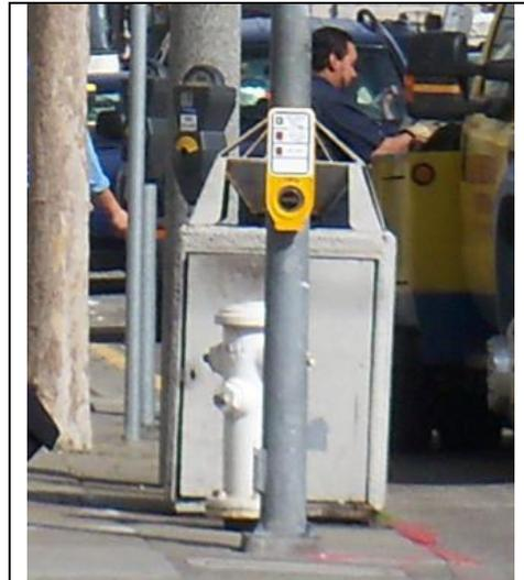
**Figure 15 - Five Intersections Are Equipped with APS**
