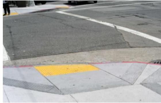
**Figure 13 – Tactile Domes Are Installed on Some Curb Ramps**
