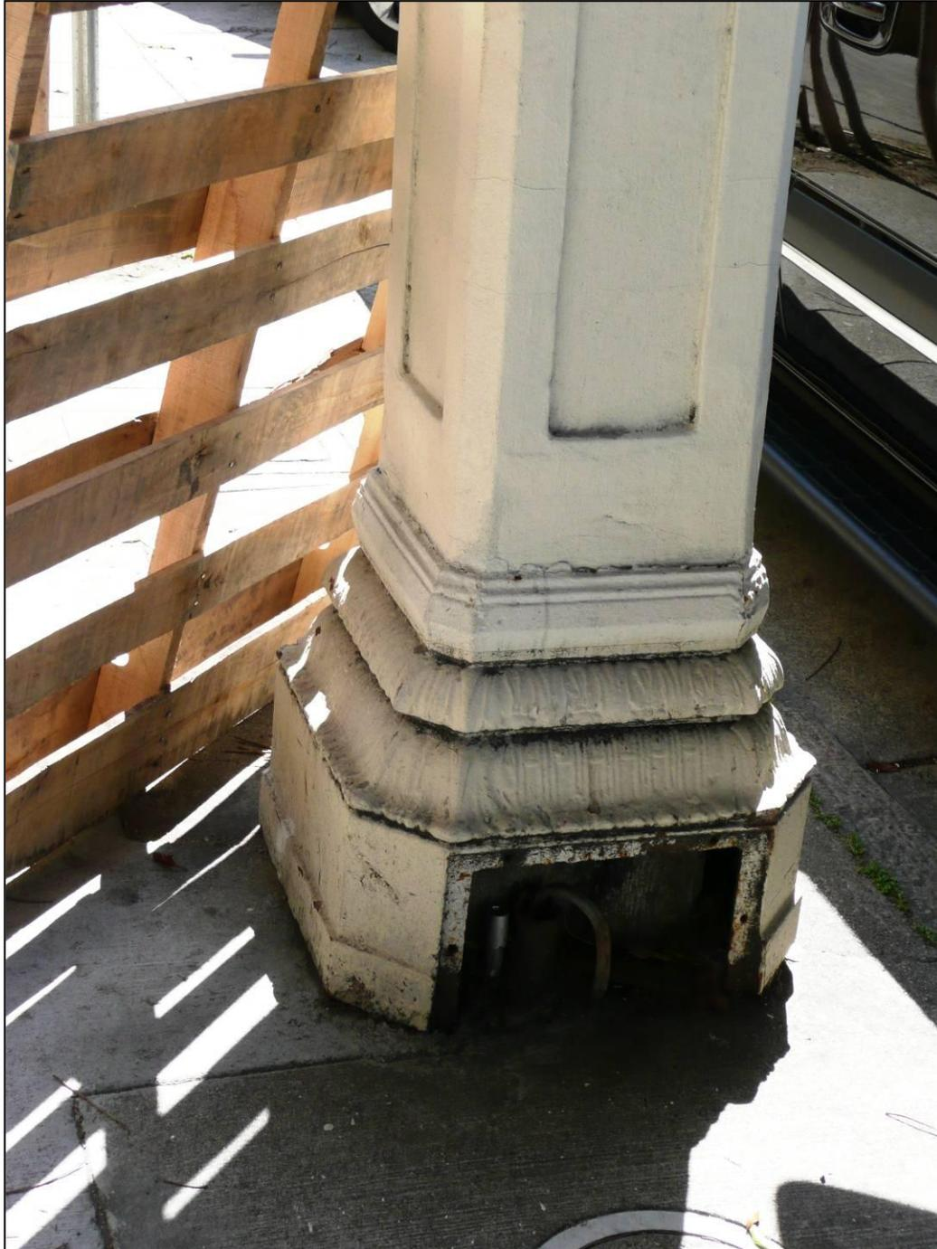
**Photograph 3: Original pole and base, missing access door, Pole 196, east side of Van Ness between Jackson and Washington, 4/1/2009.**
