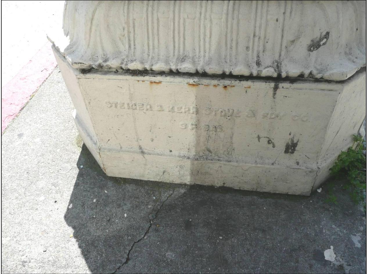
**Photograph 8:** Mark of “Steiger & Kerr Stove & Foundry Co., SF CA,” on iron replacement base access door on Pole 211, northwest corner of Van Ness Avenue and Pacific Street, 4/1/2009.
