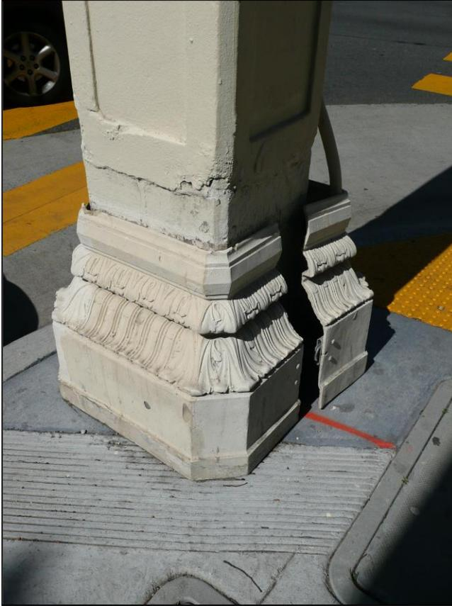
**Photograph 15a and 15b:** Example of fiberglass replacement base (this one with foliated detailing), no access doors, Pole 308, at the southeast corner of Van Ness and Bay, 4/1/2009.
