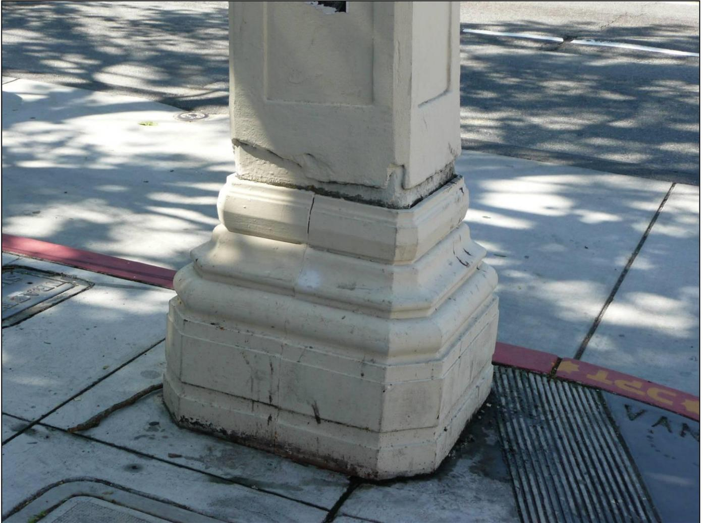
**Photograph 9: Replacement fiberglass base without foliated details or access doors, Pole 228, southeast corner of Van Ness Avenue and Vallejo Street, 4/1/2009.**
