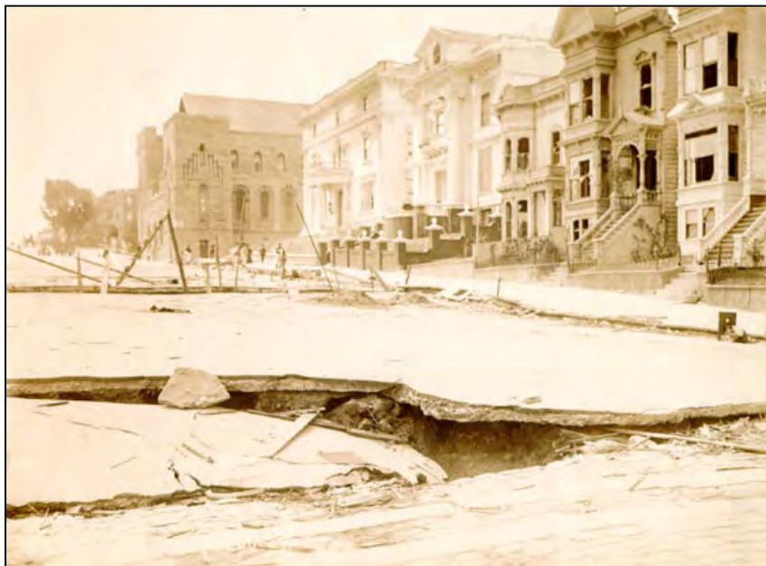
Figure 10: Earthquake Damage Along Van Ness Avenue at Vallejo Street (Area 3), 1906. While there was much damage along the avenue, a number of buildings remained structurally sound. (San Francisco History Center 1906)
