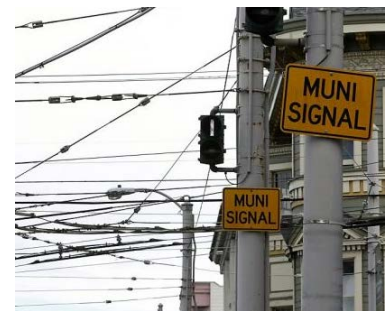
Muni Overhead Contact System (OCS) Photo credit: SFGATE
