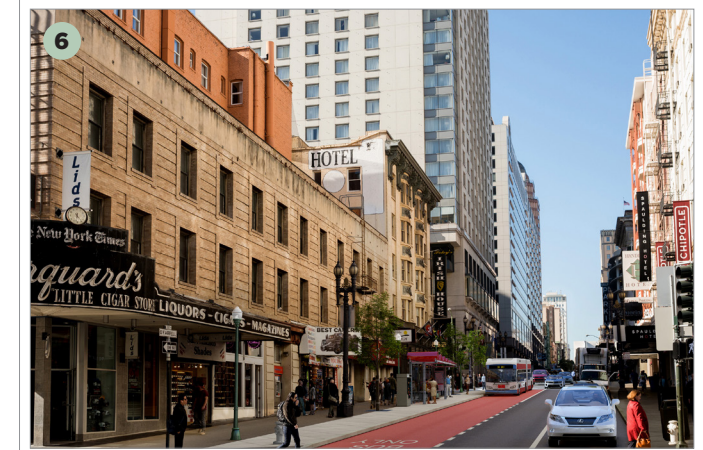
Gough to Market: Enhancements to Existing Side Lanes Colorizes existing lanes, fills existing gaps in bus lanes, improves bus flow at key intersections, and provides bus bulb-outs at high-ridership stops. Preserves curbside loading access for hotels, theaters, and stores.
