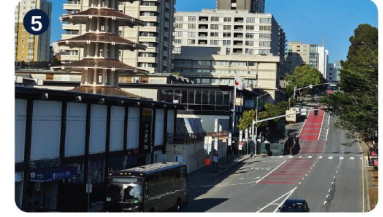
Parking garage entries, loading, and surface parking dominate the frontages
