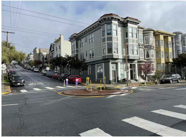
Figure 3-23. Slow Street and roundabout on Lyon St
