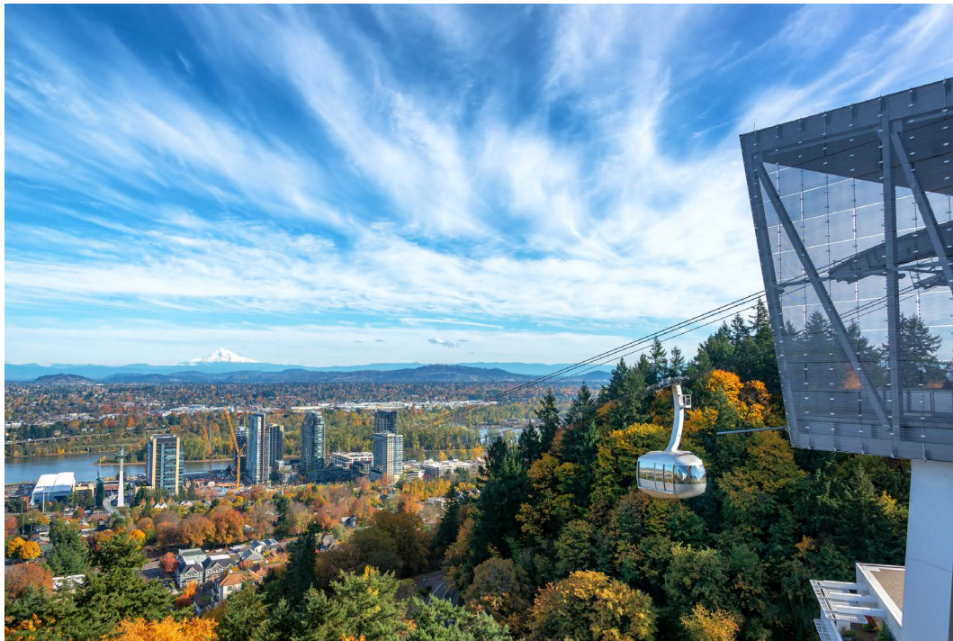
Figure A-1. Portland Aerial Tram, Portland, OR
