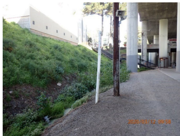
Figure 12 Southbound Platform Drainage Ditch
