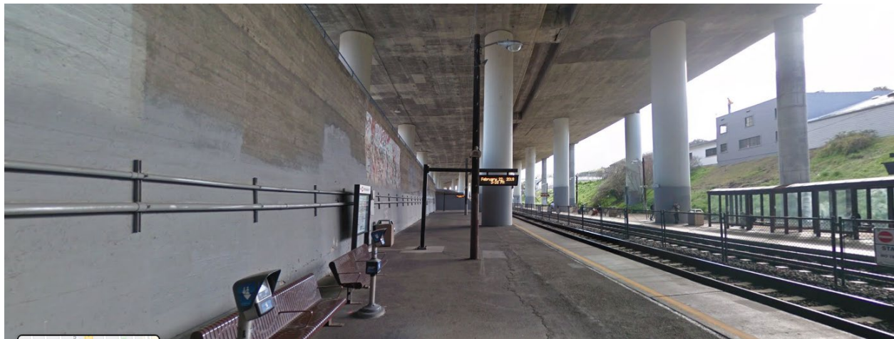
Figure 3 Northbound Platform Retaining Wall
