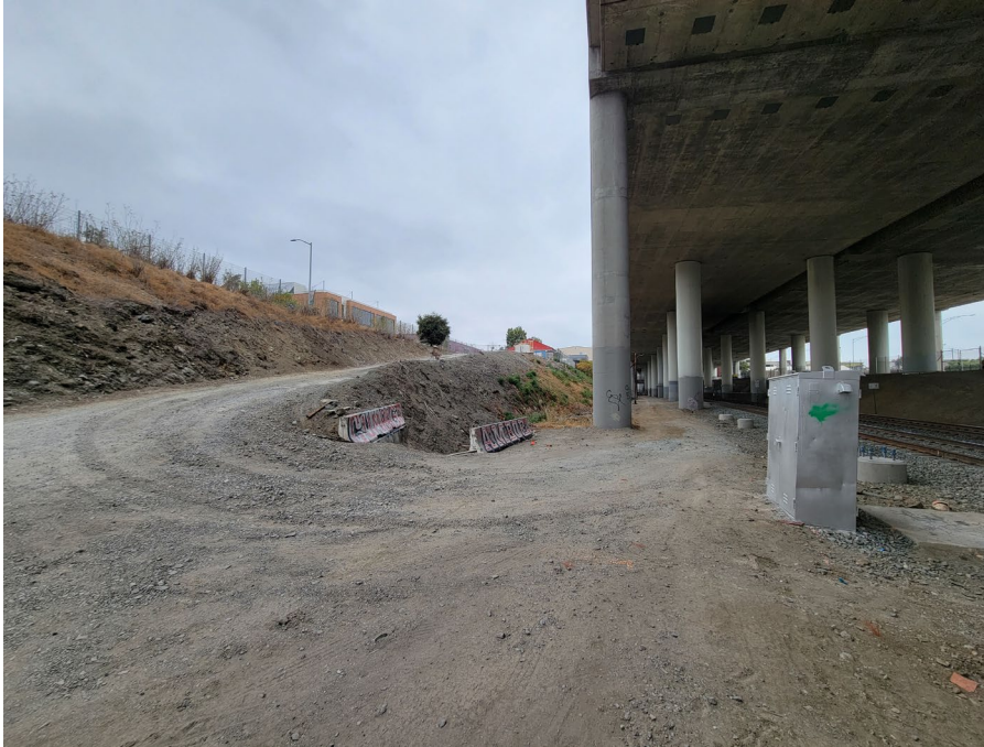
Figure 8 Southbound Platform Gravel Access Road
