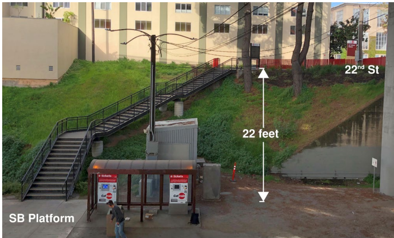
Figure 9 Southbound Platform Staircase
