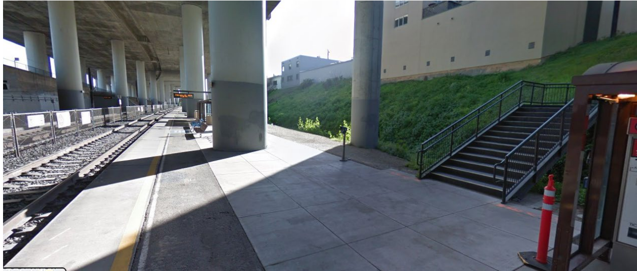
Figure 10 Southbound Platform Looking Southward from TVM
