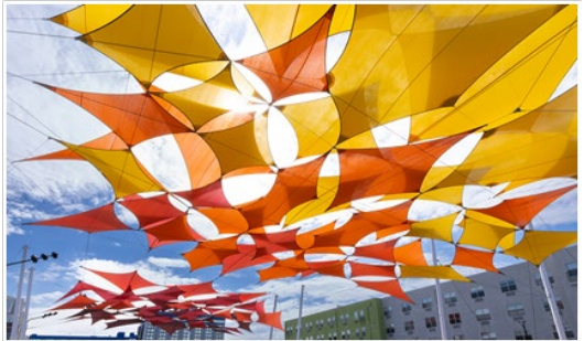
OVERHEAD SHADE STRUCTURE
