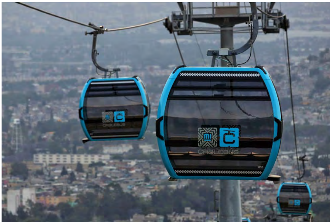
Figure A-6. Mexico City Cablebús, Mexico City, Mexico
