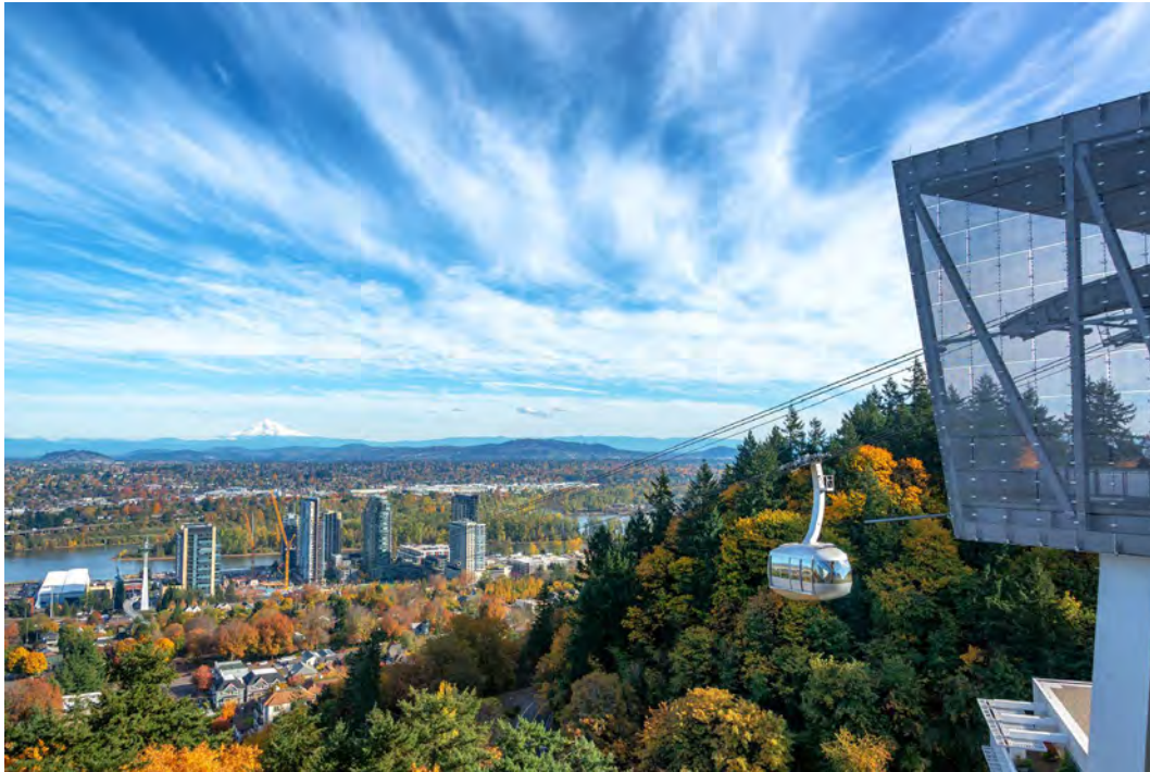
Figure A-1. Portland Aerial Tram, Portland, OR
