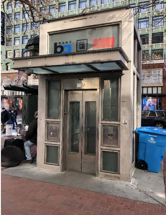
Figure 6. Street elevator at Powell St. Station, December 2021.
