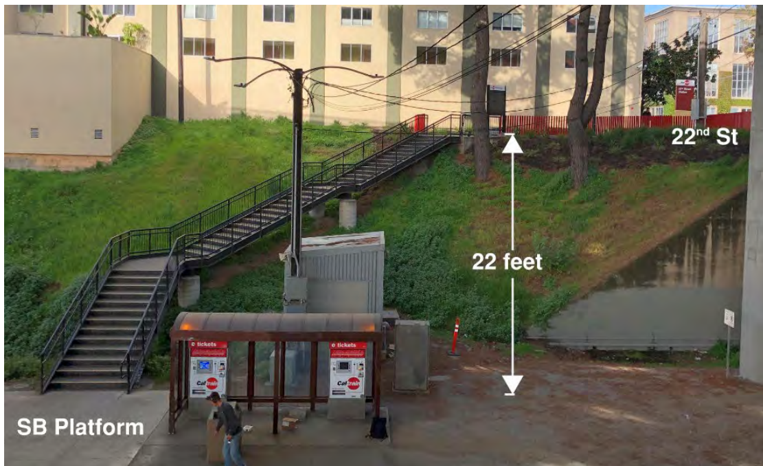
Southbound Platform Staircase
