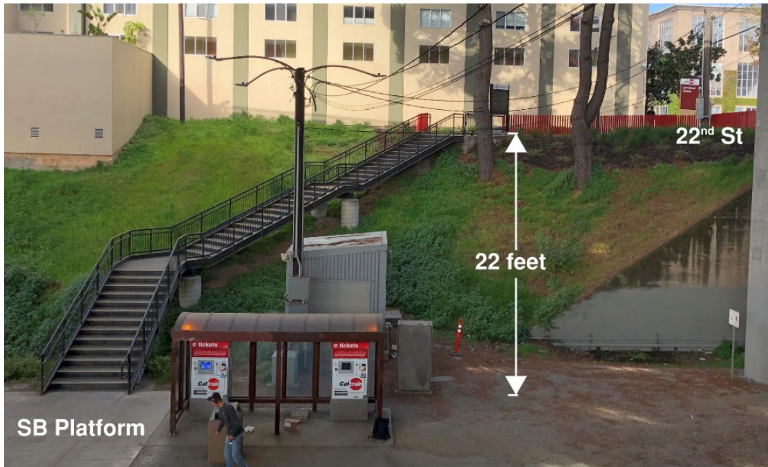
Southbound Platform Staircase
