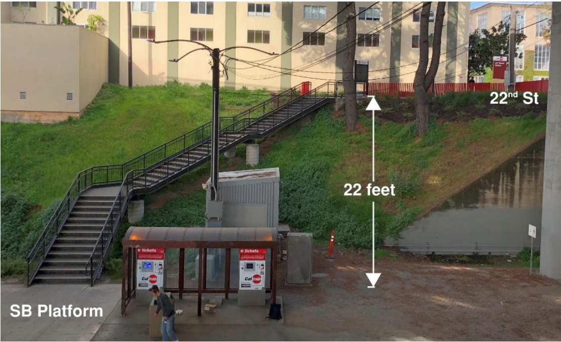
Southbound Platform Staircase
