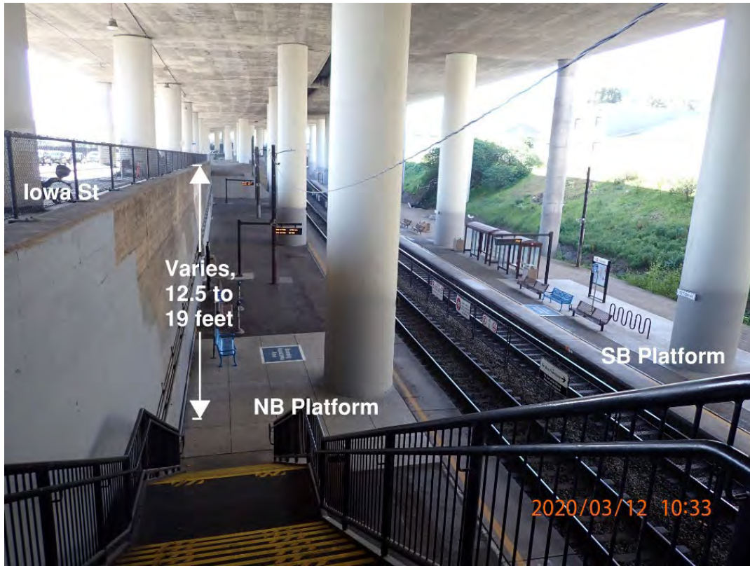
Northbound Platform, Facing South from the Top of the Staircase
