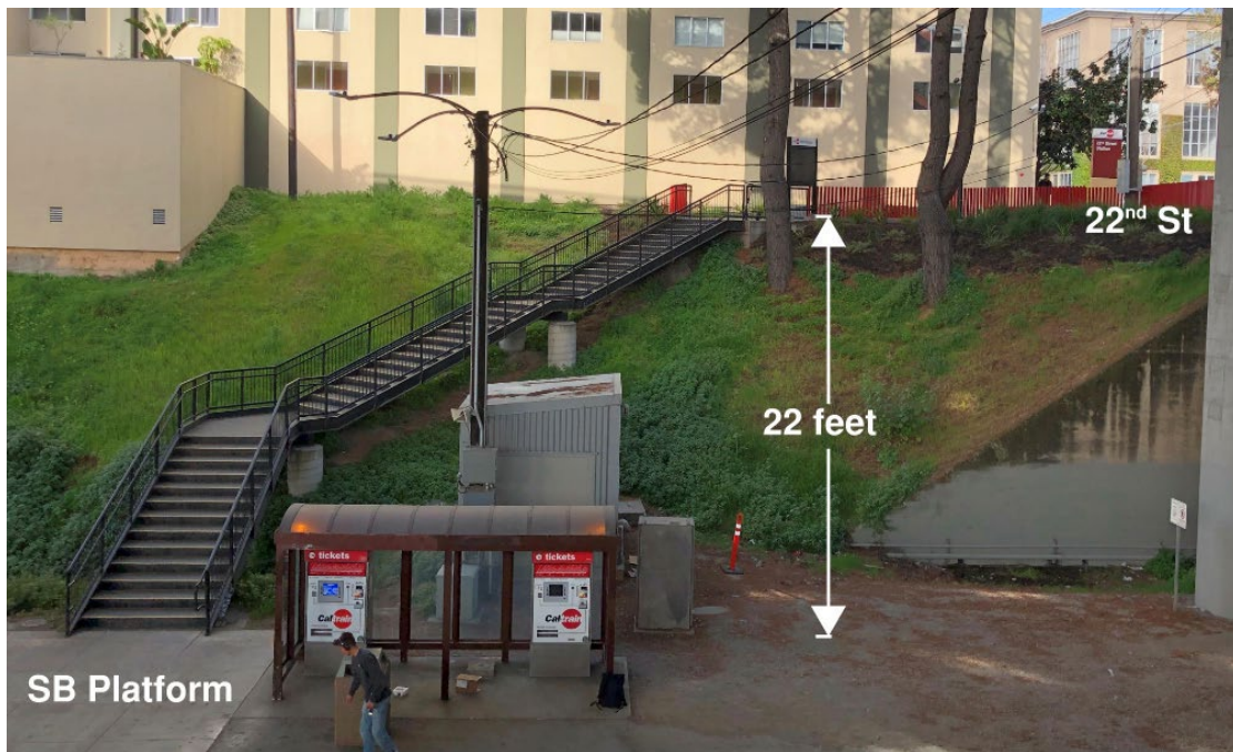
Southbound Platform Staircase
