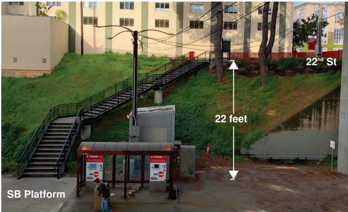
Southbound Platform Staircase
