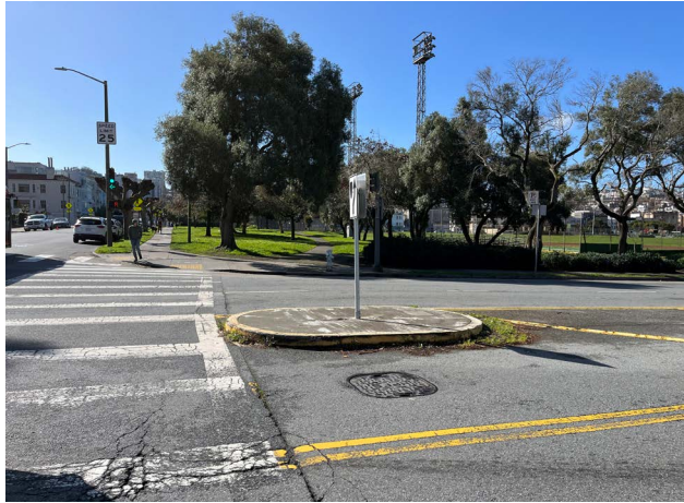
Figure 3-15. Traffic calming median on Bay Street
