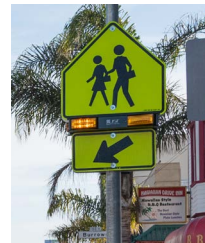
Flashing pedestrian beacon
