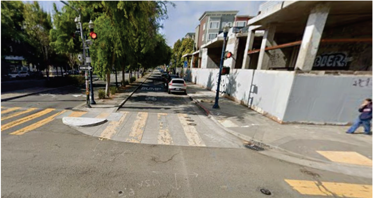
Figure 5. Octavia northbound local lane at Oak Street. This crossing is proposed to be raised (to the side median) in order to calm traffic and improve the pedestrian crossing experience (regardless of what is happening, or not, with the adjacent freeway parcel properties).
