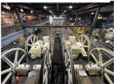
Figure K: Completed Gearbox Works at Cable Car Barn and Powerhouse, January 2023
