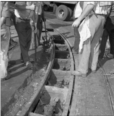
Figure L: Cable Car Track Repairs at Washington and Powell Streets, October 1979
