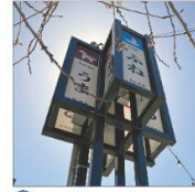
12 reinstall (5) lamp posts
