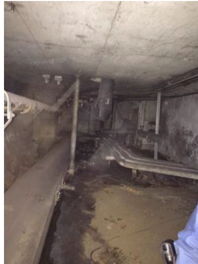
Relocate existing utilities and reconfigure platform areas
