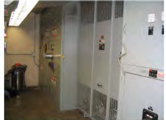
Medium Voltage Service Entrance Switchgear, 2.5 MW Medium Voltage Transformer and 480 V Switchboard
