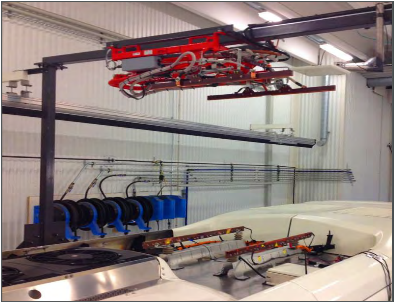
Figure 3-1. Inverted Pantograph and Charge Rails
