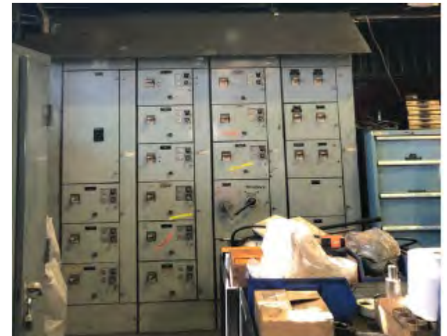
Motor Control Center (MCC)
