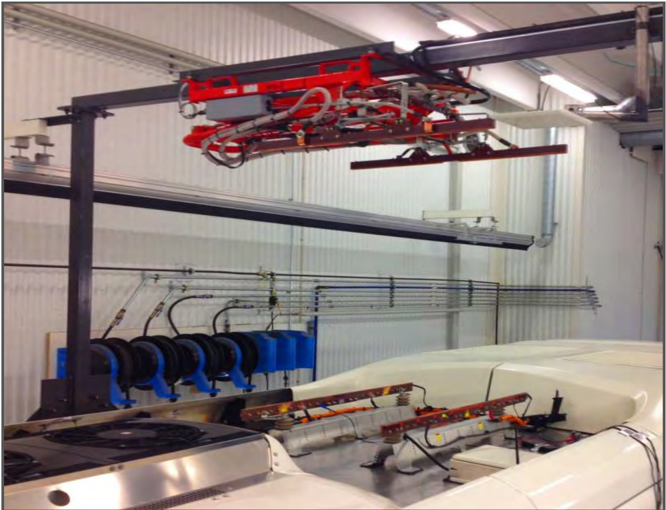
Figure 3-1. Inverted Pantograph and Charge Rails
