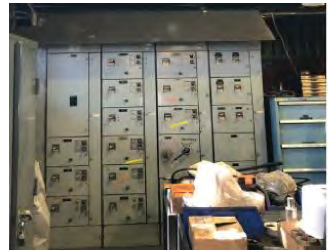
Motor Control Center (MCC)
