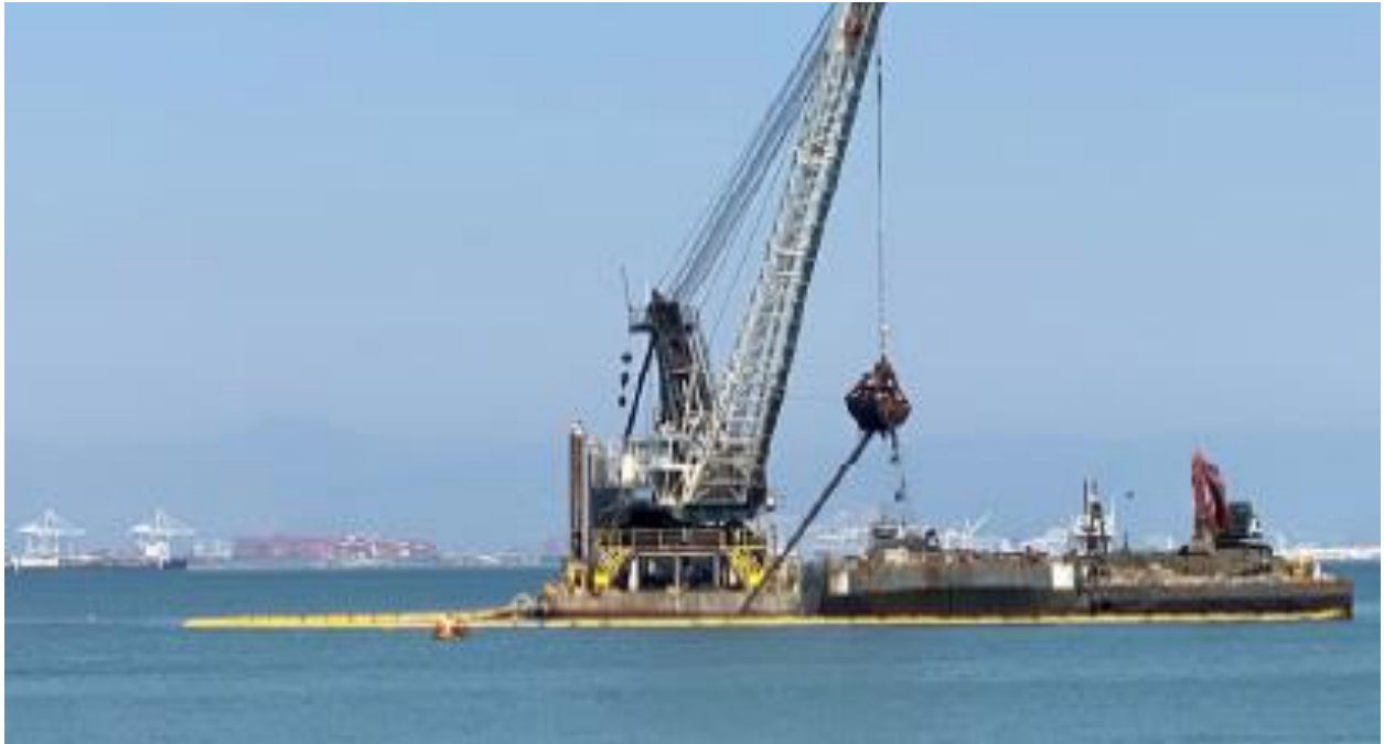
Figure 7: Dredge using 6 cy bucket to remove full pile from MBFL dredge area prior to NUAD dredging, Sept 4, 2020.
