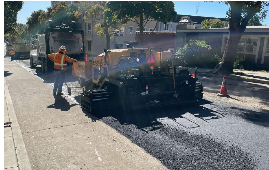
Similar recent Prop K-funded SFPW paving work on Laguna Street
