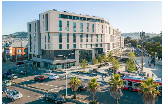
Transportation Authority funding helped construct a new public plaza at BART's Balboa Park Station.
