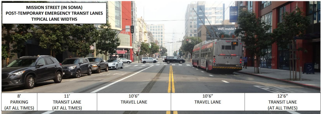
Figure 2: Cross-sections: Previous (above) and Current/Proposed (below)
