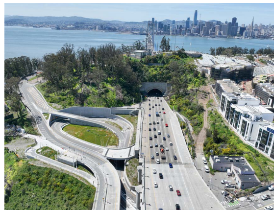
The Southgate Realignment project opened for use in Spring 2023.
