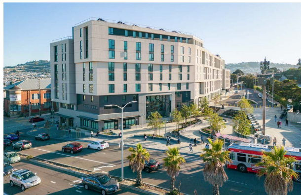
Transportation Authority funding helped construct a new public plaza at BART's Balboa Park Station.
