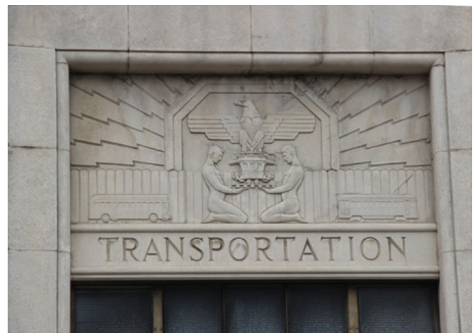
FIGURE 3-28: PANEL ABOVE ON EAST FAÇADE ENTRANCE
