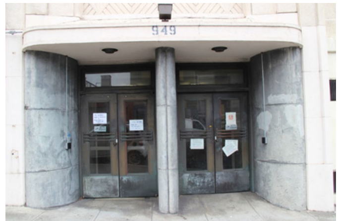
FIGURE 3-27: ENTRANCE PAVILION DOORS
