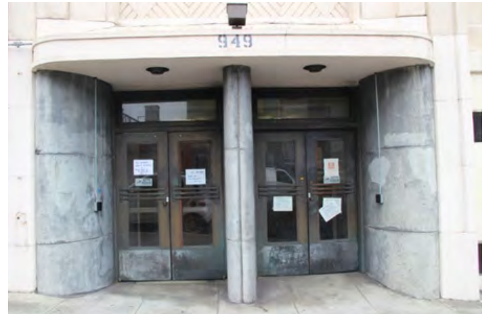
FIGURE 3-27: ENTRANCE PAVILION DOORS
