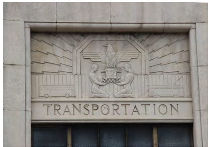
FIGURE 3-28: PANEL ABOVE ON EAST FAÇADE ENTRANCE
