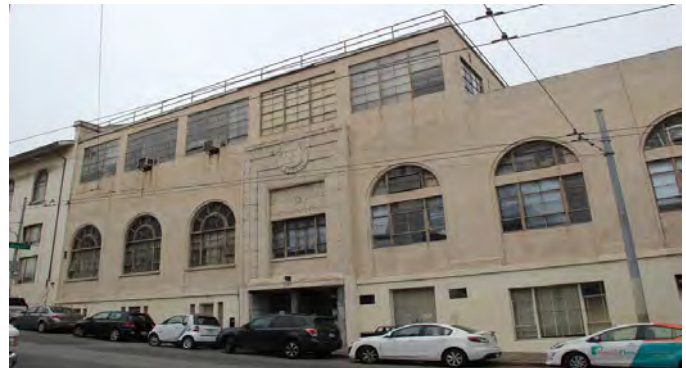
FIGURE 3-24: 1914 MAINTENANCE WING ADDITION ART DECO
