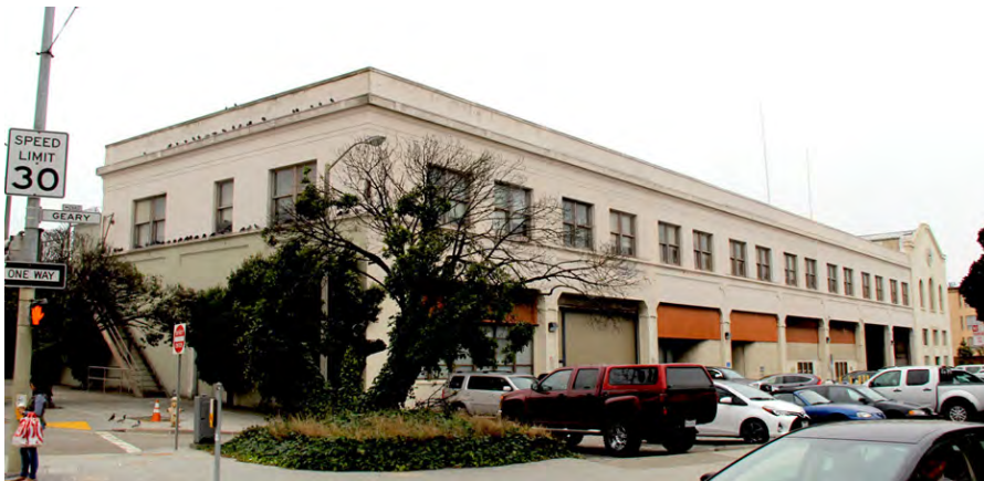
FIGURE 3-21: PRESIDIO TROLLEY COACH DIVISION OFFICE BUILDING
