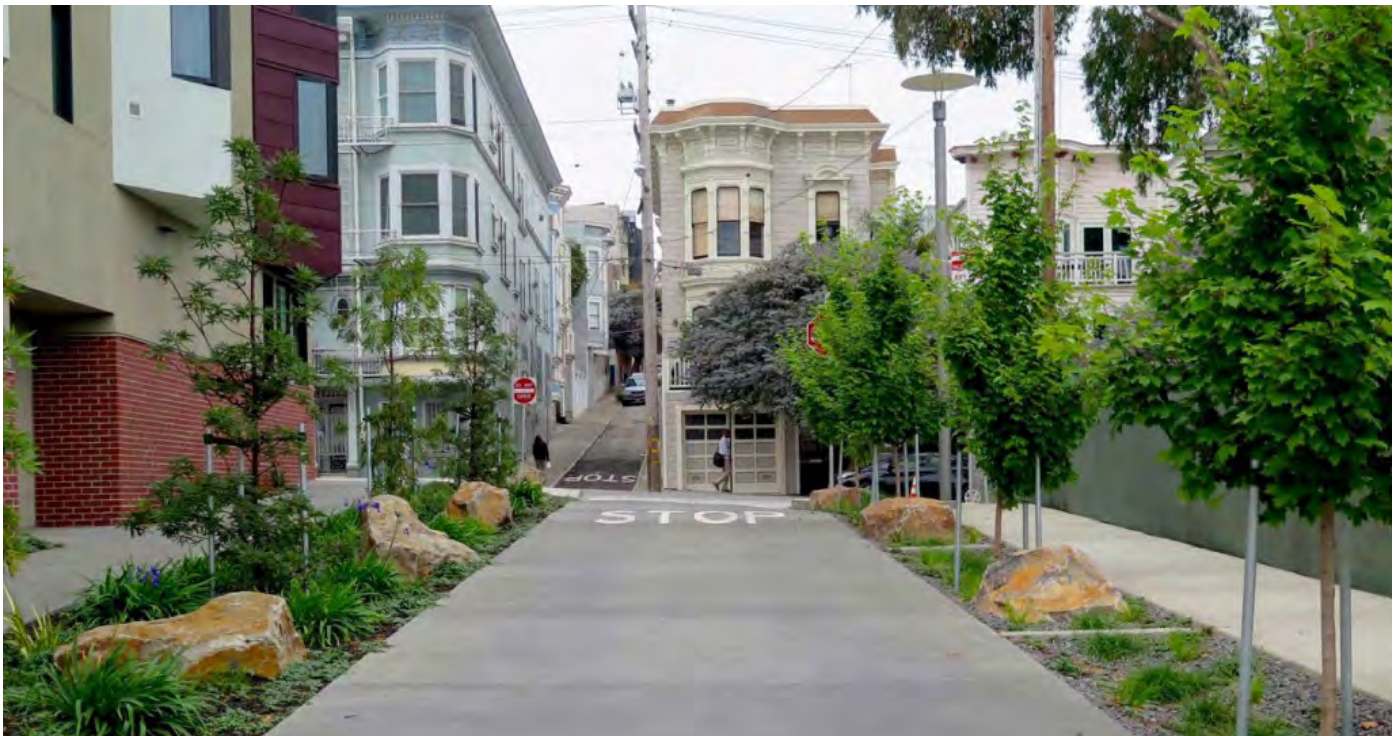
FIGURE 4-2: BIORETENTION ALONG STREET AND SIDEWALKS
