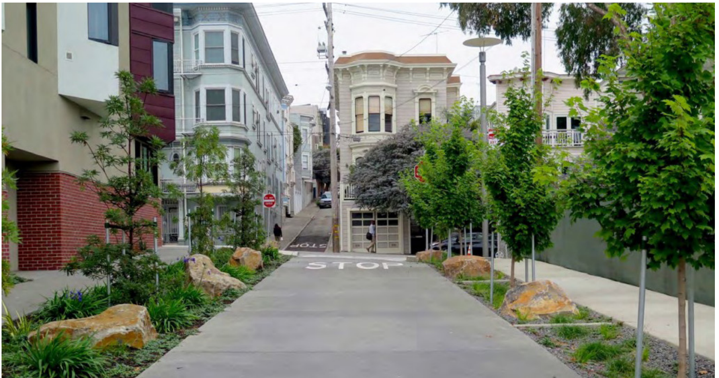
FIGURE 4-2: BIORETENTION ALONG STREET AND SIDEWALKS
