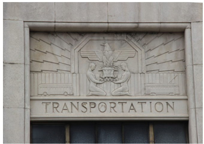
FIGURE 3-28: PANEL ABOVE ON EAST FAÇADE ENTRANCE
