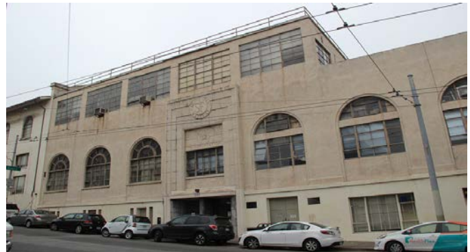
FIGURE 3-24: 1914 MAINTENANCE WING ADDITION ART DECO
