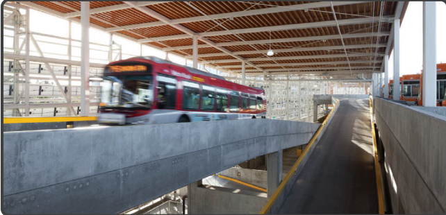
Circulation Ramps: Main circulation area that allows vehicles to move up and down between floors.
