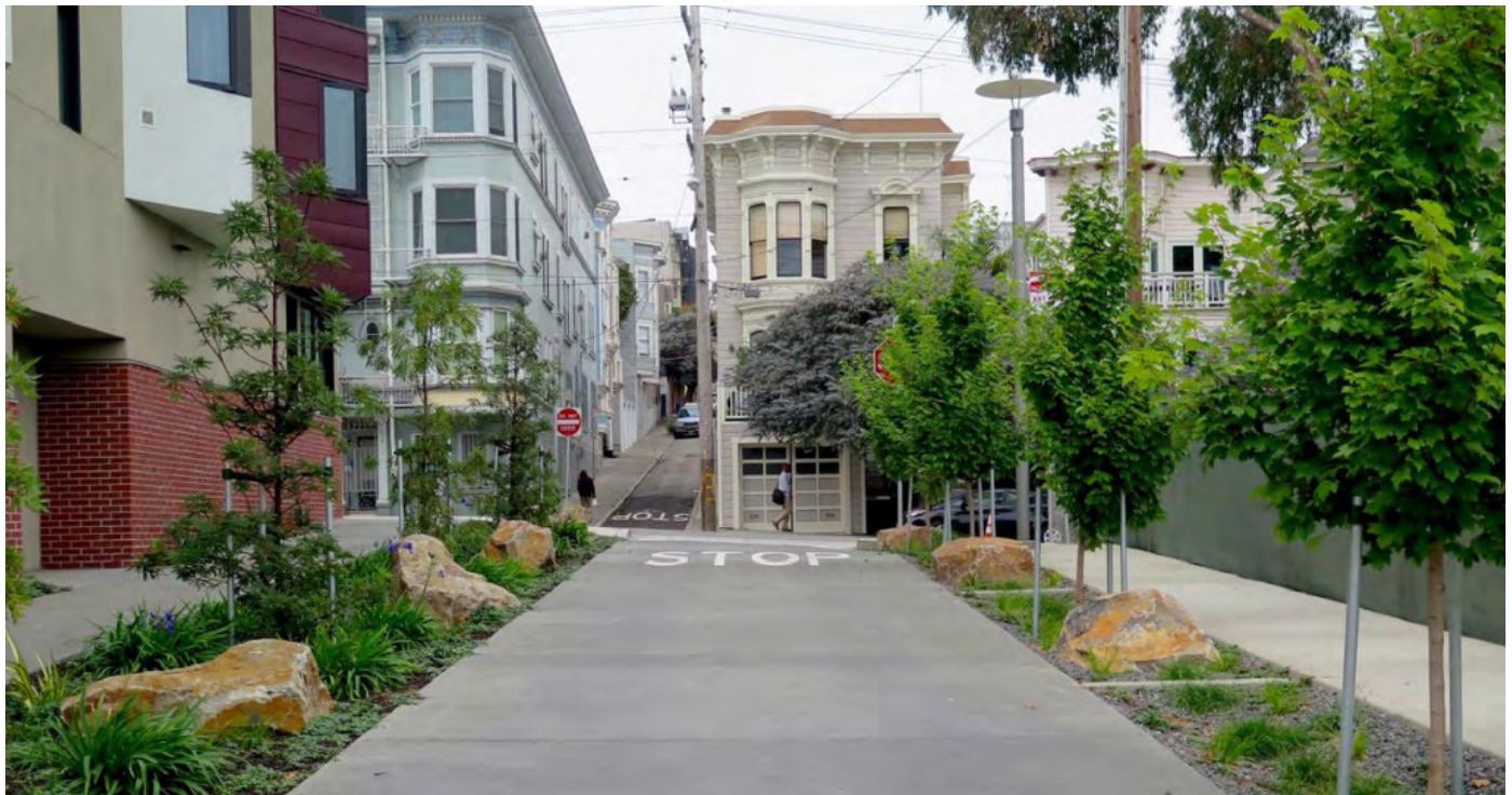
FIGURE 4-2: BIORETENTION ALONG STREET AND SIDEWALKS
