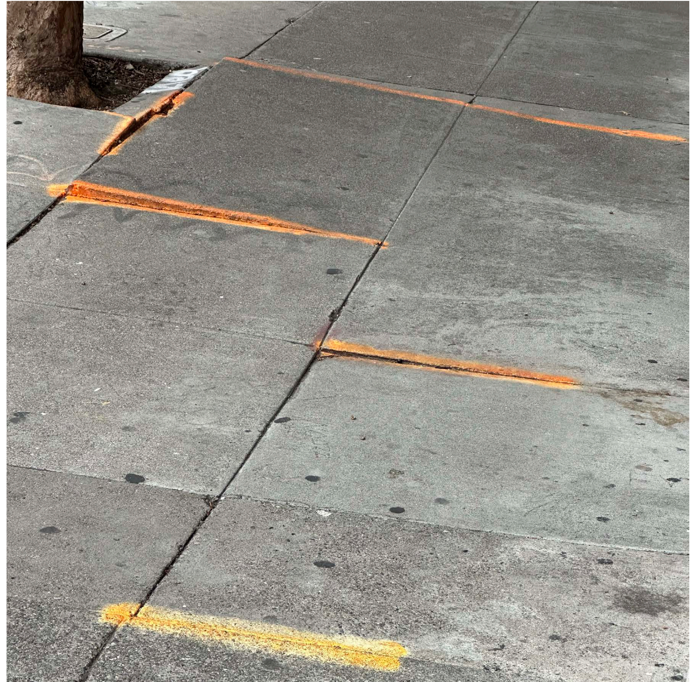
Side way cracks on Valencia at 14th Street
