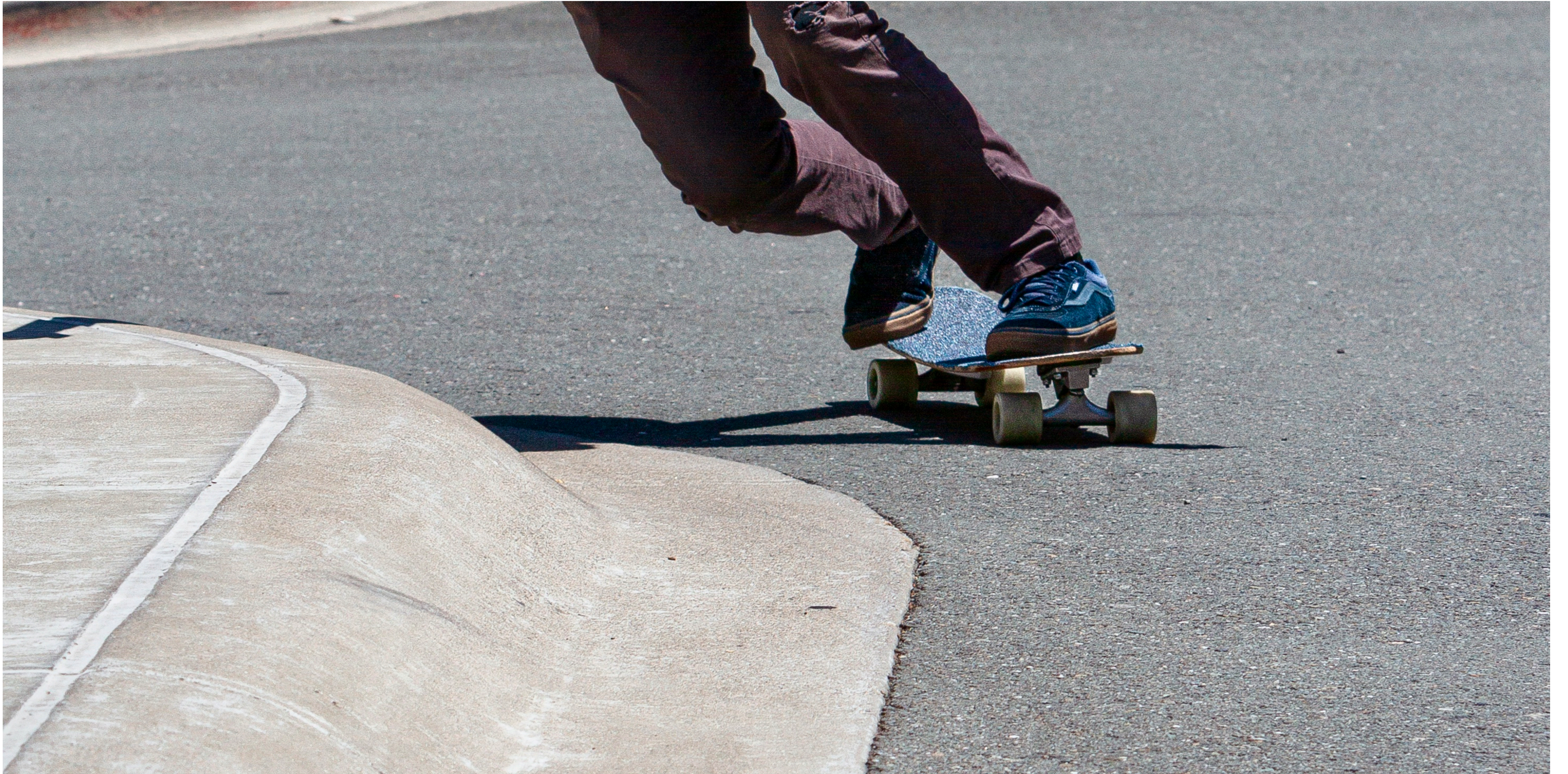
Rolled curb in Oakland
