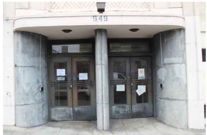
FIGURE 3-27: ENTRANCE PAVILION DOORS
