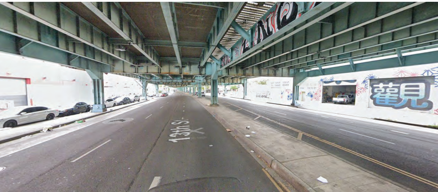
13 th Street between South Van Ness Avenue and Folsom Street, facing east
