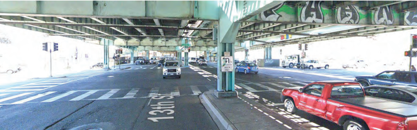
13 th Street at South Van Ness Avenue, facing west
