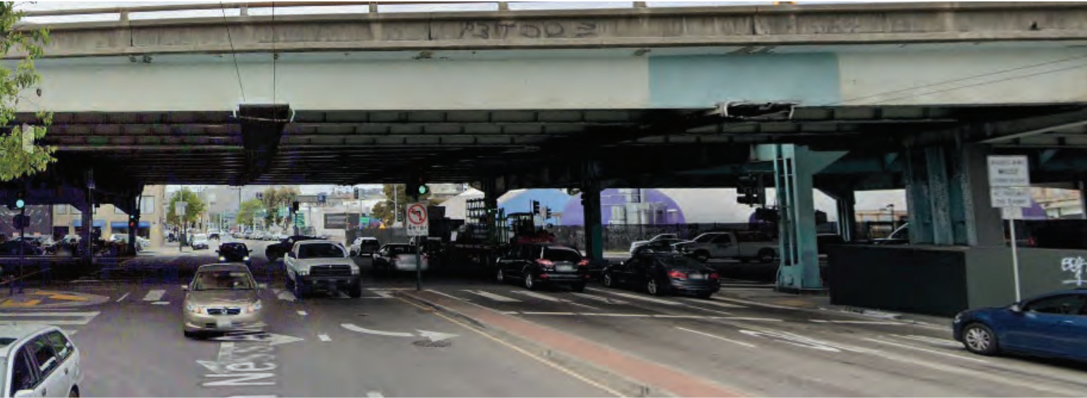
13 th Street at South Van Ness Avenue, facing south
