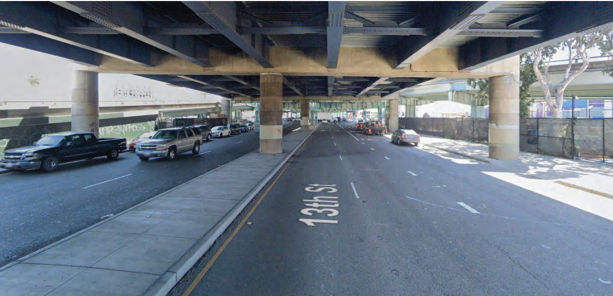
13 th Street between Otis Street/Mission Street and South Van Ness Avenue, facing east
