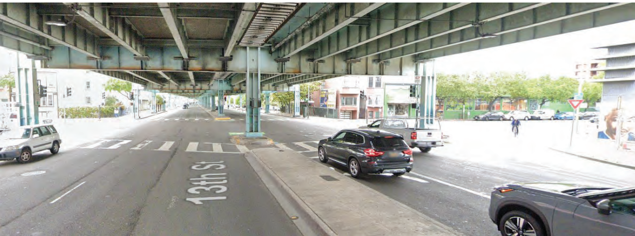
13 th Street at Folsom Street, facing east
