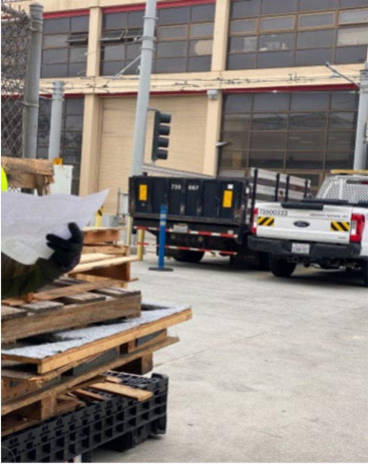
Photo 12: Existing Green Building Outside
