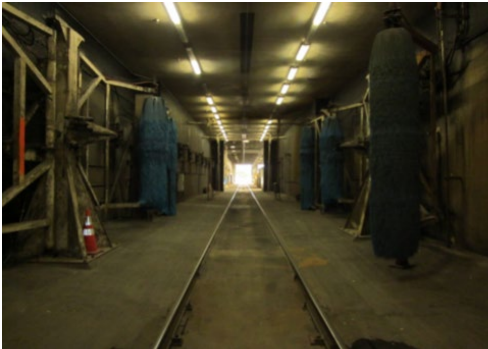
Photo 14: Existing Green Car Wash Facility
