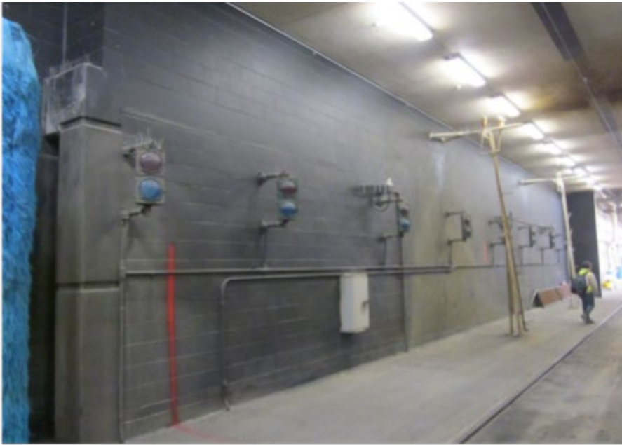
Photo 15: Existing Green Car Wash Facility
