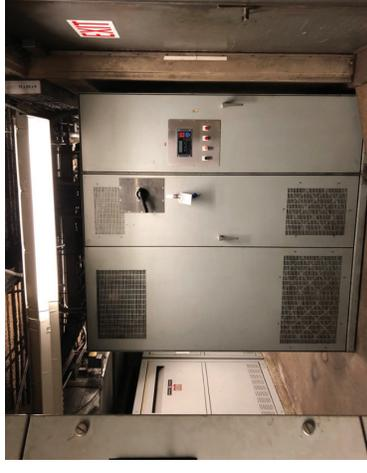
DC Motor Drive Speed Variator Power Unit Model 6V600F3036 – 510 HP, 480 Volts, 680 Amps, 60 Hertz, 3 Phase DC3064R Power Unit
