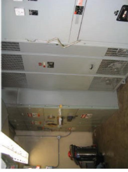
Medium Voltage Service Entrance Switchgear, 2.5 MW
