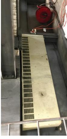
*Non-Functioning Fin Coil Unit in Cable Car Pits*
