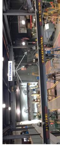
*Ventilation Equipment Mounted on Structural Support at First Floor Mezzanine*
