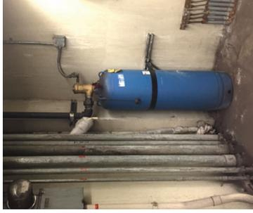
*Halon Cylinder in Electrical Equipment Room Prior to September 9, 2021 Discharge*
