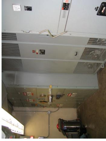
Medium Voltage Service Entrance Switchgear, 2.5 MW Medium Voltage Transformer and 480 V Switchboard
