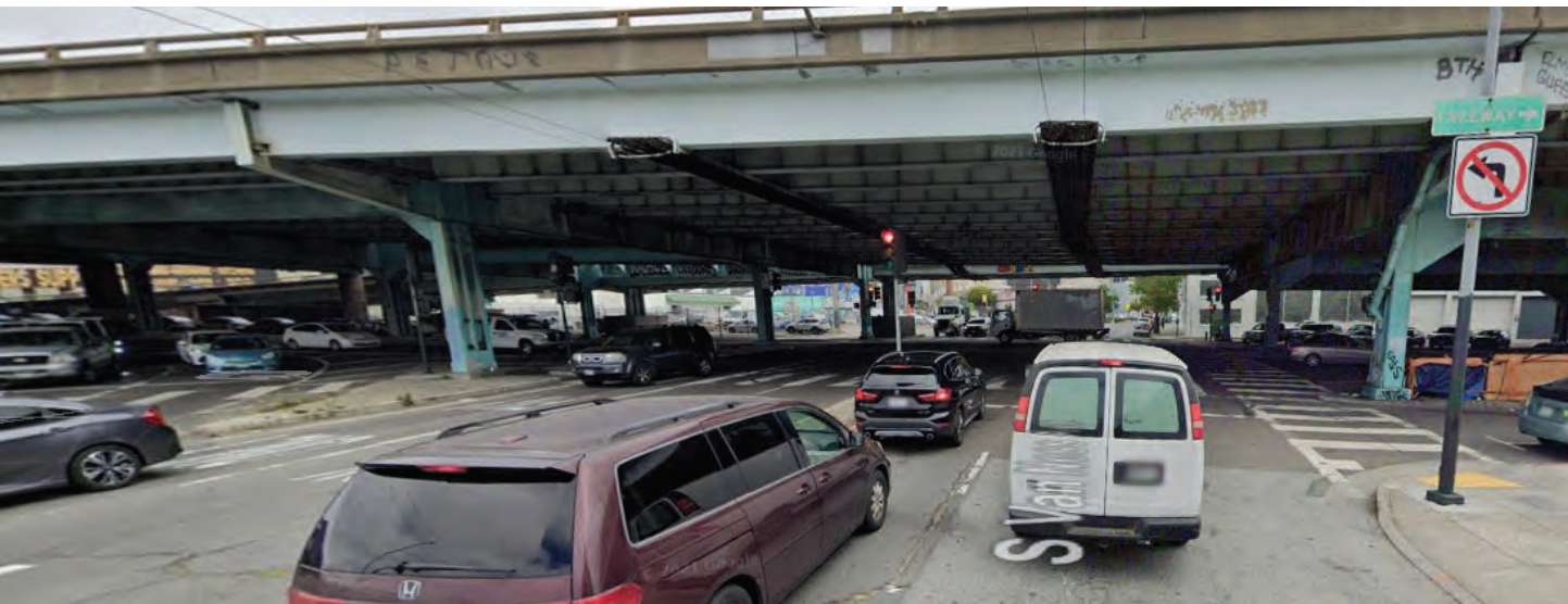
13 th Street at South Van Ness Avenue, facing north
