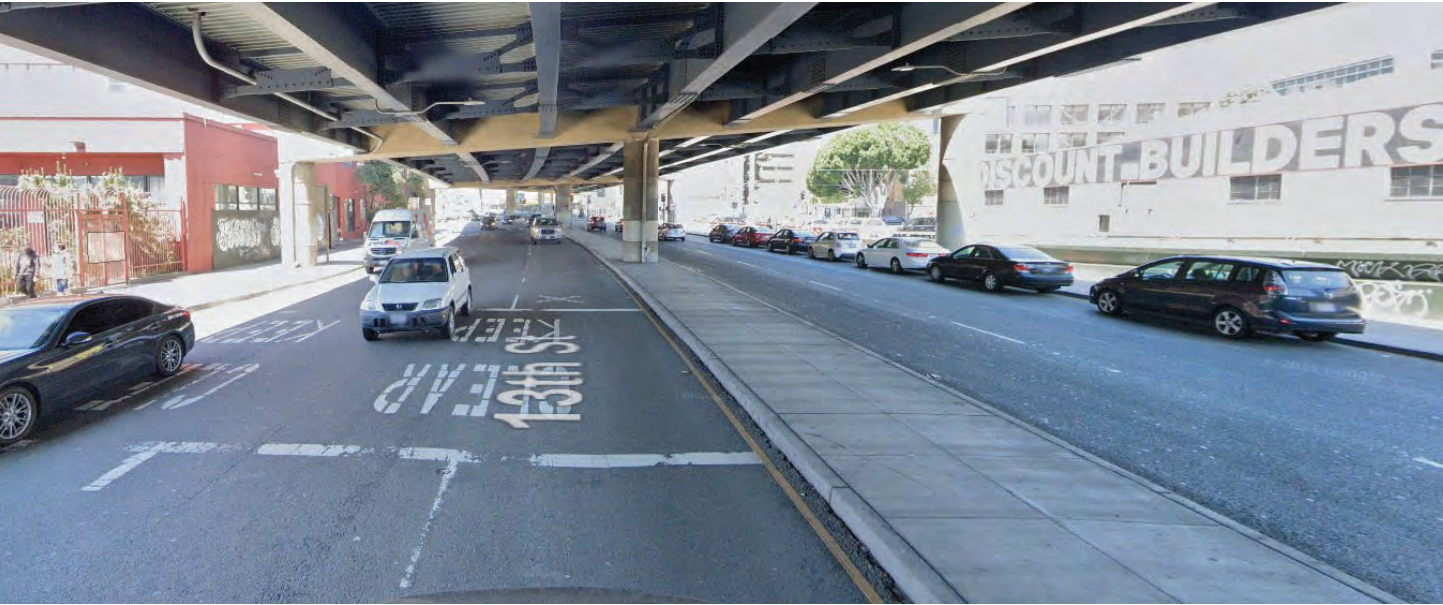
13 th Street between Otis Street/Mission Street and South Van Ness Avenue, facing west
