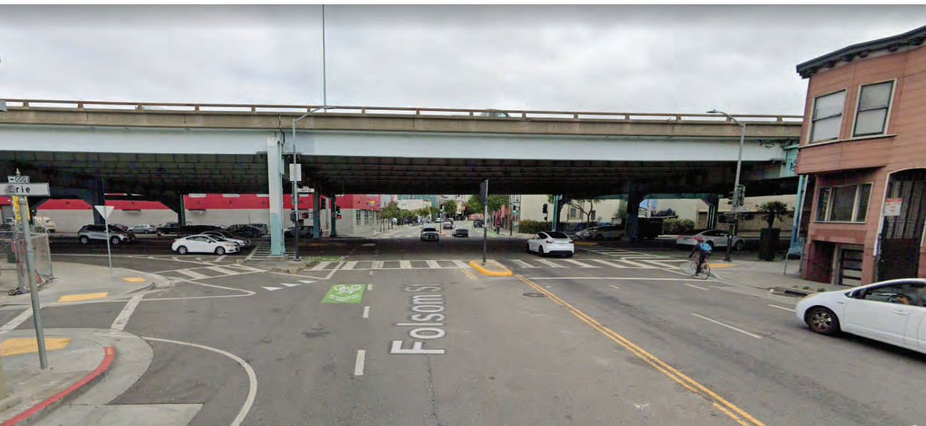
13 th Street at Folsom Street, facing north
