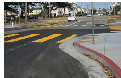
Curb Bulbout with newly painted crosswalks
