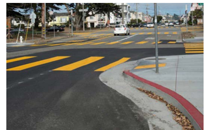
Curb Bulbout with newly painted crosswalks
