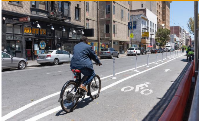
Paint, signs, and delineators
