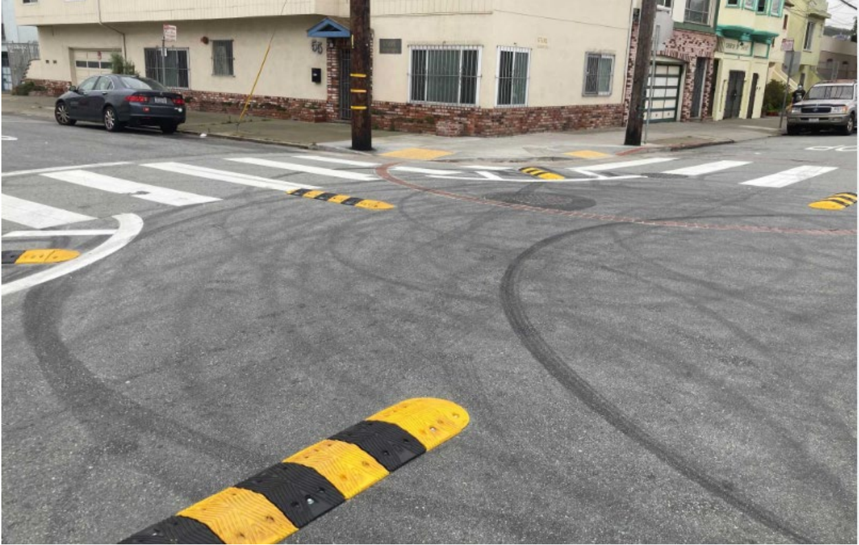
Centerline and corner hardening w/paint and rubber speed humps (Plymouth Ave and Sadowa St)
