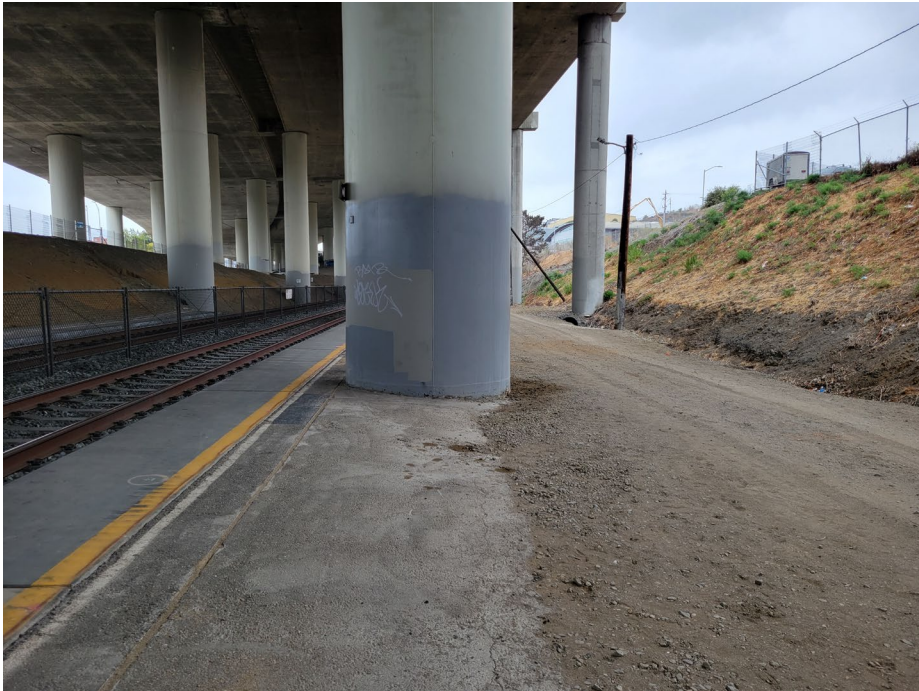
Figure 13 Southbound Platform Circulation Obstruction by I-280 Column
