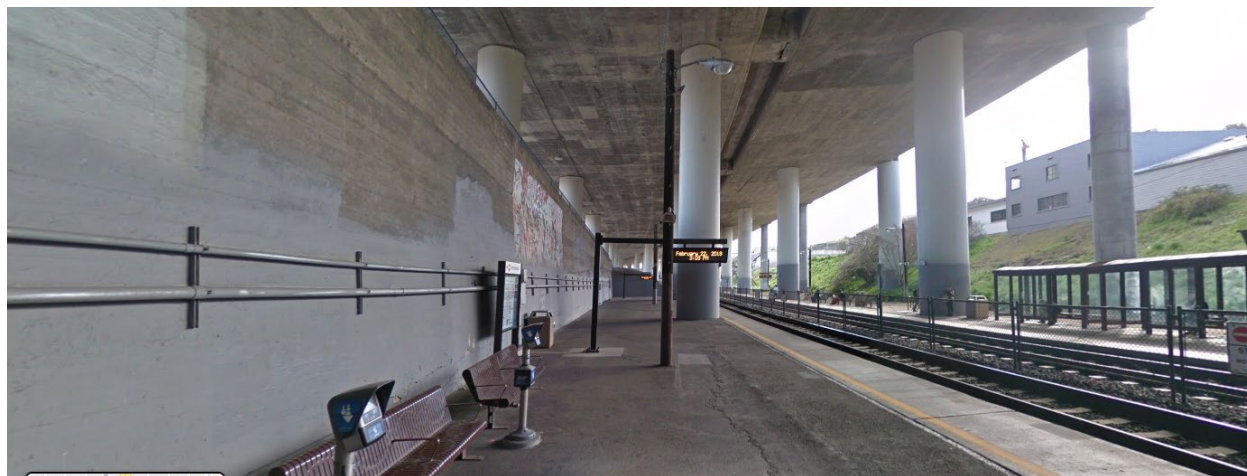
Figure 3 Northbound Platform Retaining Wall
