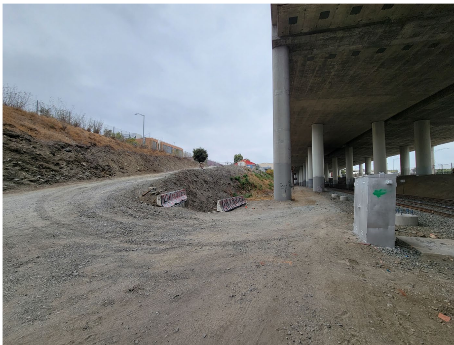
Figure 8 Southbound Platform Gravel Access Road
