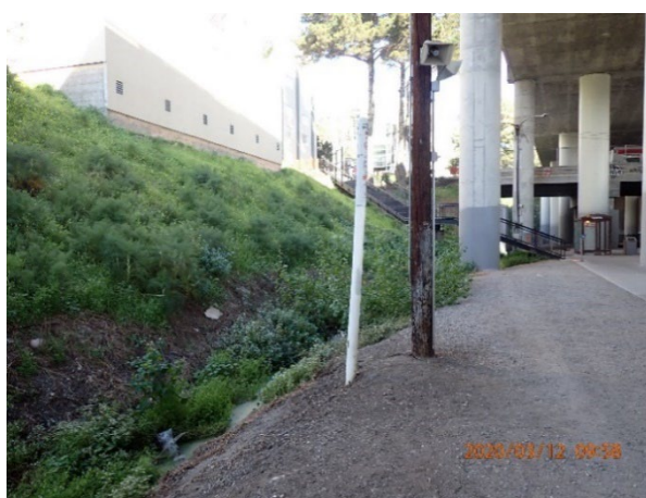
Figure 12 Southbound Platform Drainage Ditch
