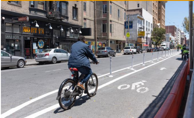
Paint, signs, and delineators
