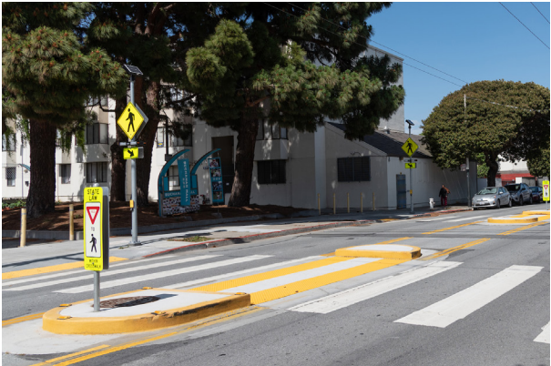
This midblock crosswalk on Fulton Street uses concrete islands that force drivers to slow down to navigate.
