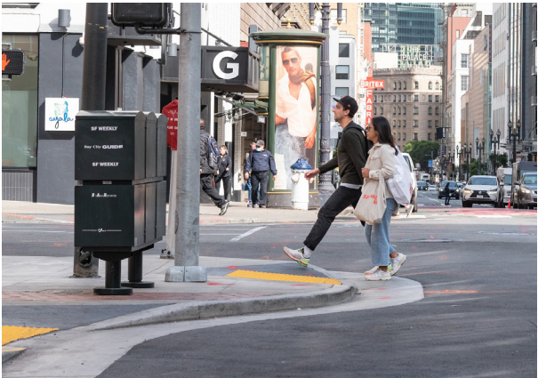
A concrete bulb-out (also known as a curb extension) on Geary Boulevard.
